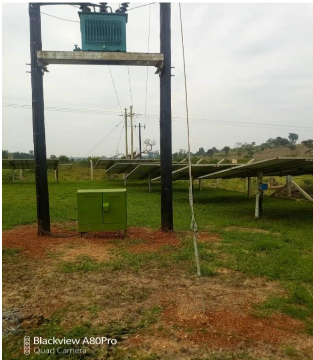
Figure 4: solar PV-grid system under study.
