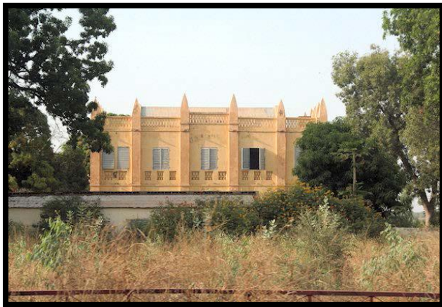
Plate, 22, e: Neo-Sudanese Style of office building at Segou, Mali
